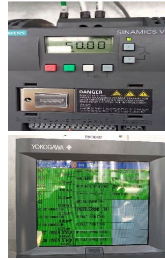
GT#12 #11 CEMS Calibration, Terminal Tighten, filter replacement, sensor cleaning
