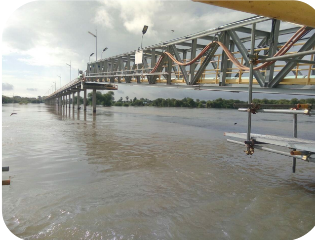
Water Pipeline (Intake & Discharge)
