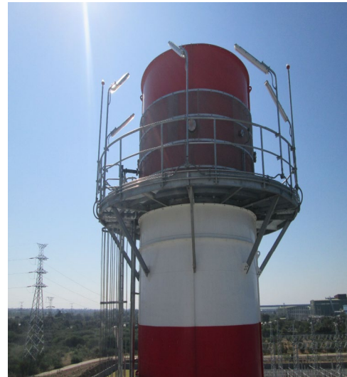
GT#12 #11 CEMS Calibration, Terminal Tighten, filter replacement, sensor cleaning
